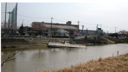
Kitakami Canal and Ishinomaki Technical High School: Ishinomaki Technical High School was inundated above the floor level by a tsunami running up the canal. The pier which the boat club had used was also destroyed.
